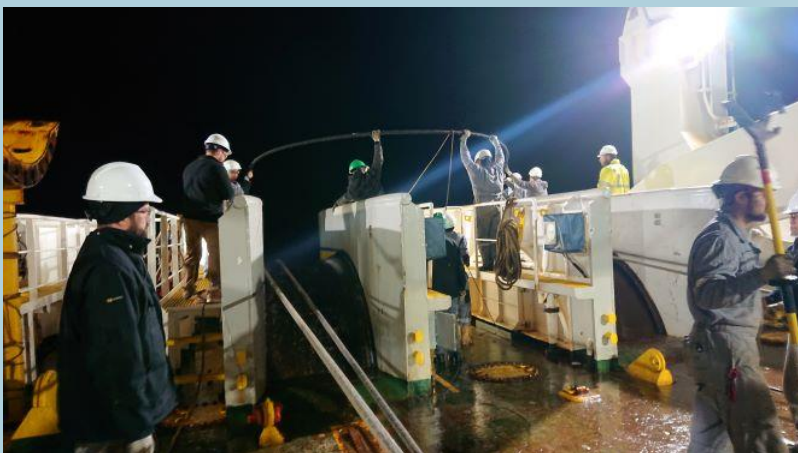
Fig. 3 The final bight crown of the Havfrue cable leaves the vessel
